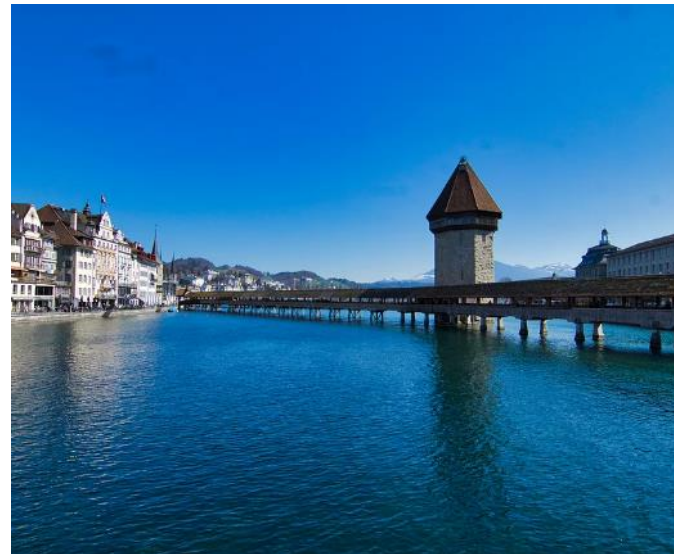
Chapel Bridge and Water Tower
